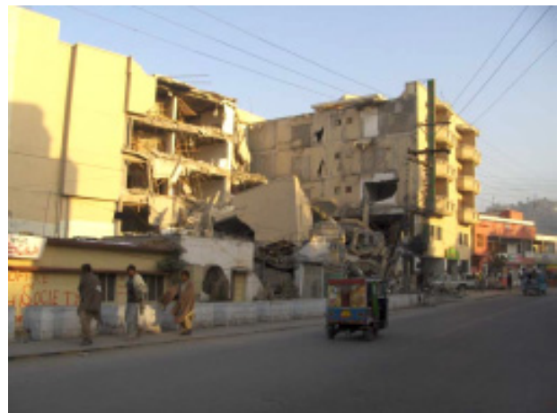
Slika 9. Podrt 5-nadstropni hotel v mestu Domel pri Muzaffarabadu Figure 9. Collapsed 5-floor hotel in Domel near Muzaffarabad
